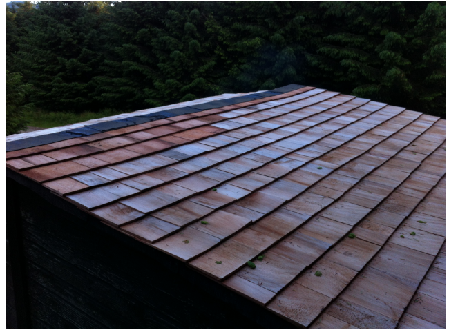
The new cedar shingle roof fits well with the woodland setting
