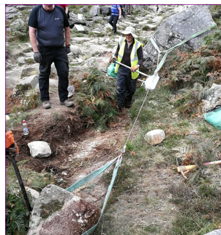
Winching rocks into place
