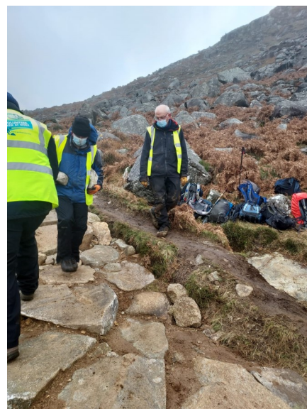
Putting the finishing touches to the track in Glendalough
