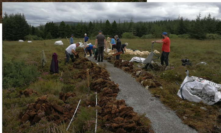
Laying a track over wool
