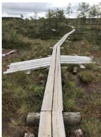
3. A duckboard trail in a heavy use area. Note the crossing points for all terrain vehicles.
