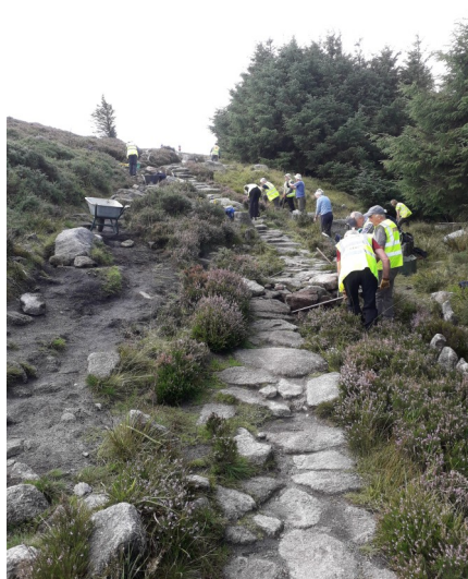
MMDW volunteers at Ticknock
