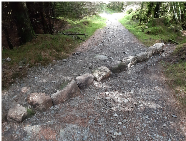
Repairing the existing gravel path at Drumgoff with water bars
