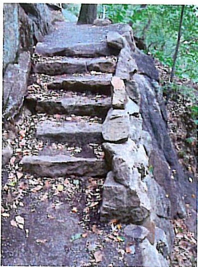
An example of buttress walls and steps clinging close to a large boulder.
