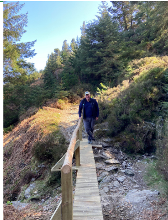
The completed Maulin foot bridge
