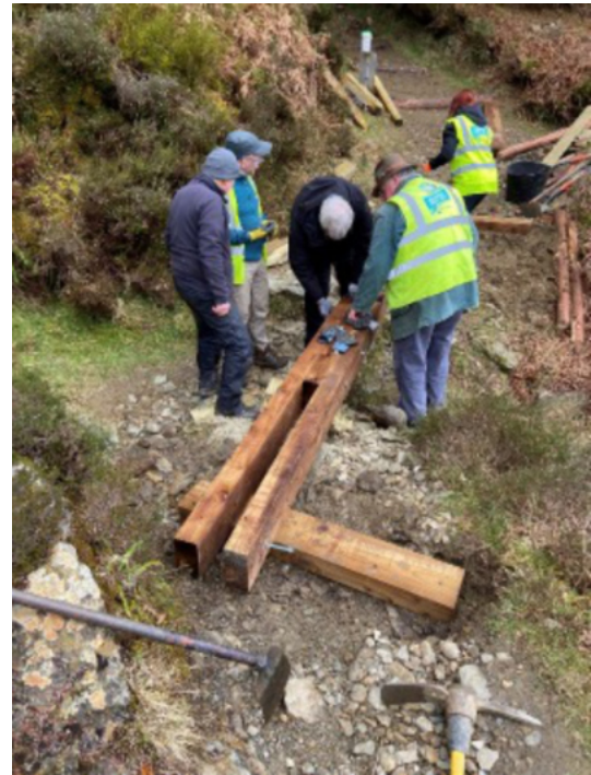
MMDW constructing a simple timber bridge on the Maulin Loop Trail
